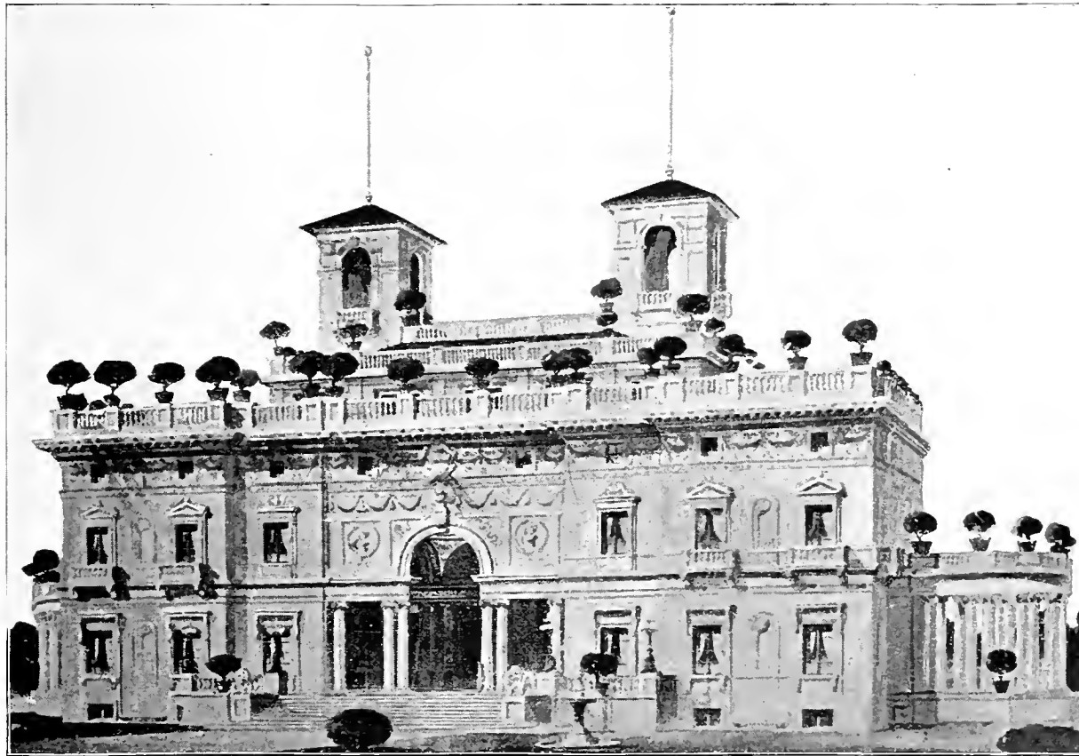
NEW YORK STATE BUILDING. — Designed by C. F. McKim of McKim, Mead, & White, New York. It is 106x214 feet, and is the most costly of the State buildings. It is 96 feet high. On the roof is a double-terraced garden of rare and beautiful plants, sheltered by ample awnings. The building is noticeable for its uniqueness, and represents a palatial Italian villa. The construction and decoration, within and without, are on a very elaborate and expensive scale, well fitting it to be the headquarters of "the Empire State."
