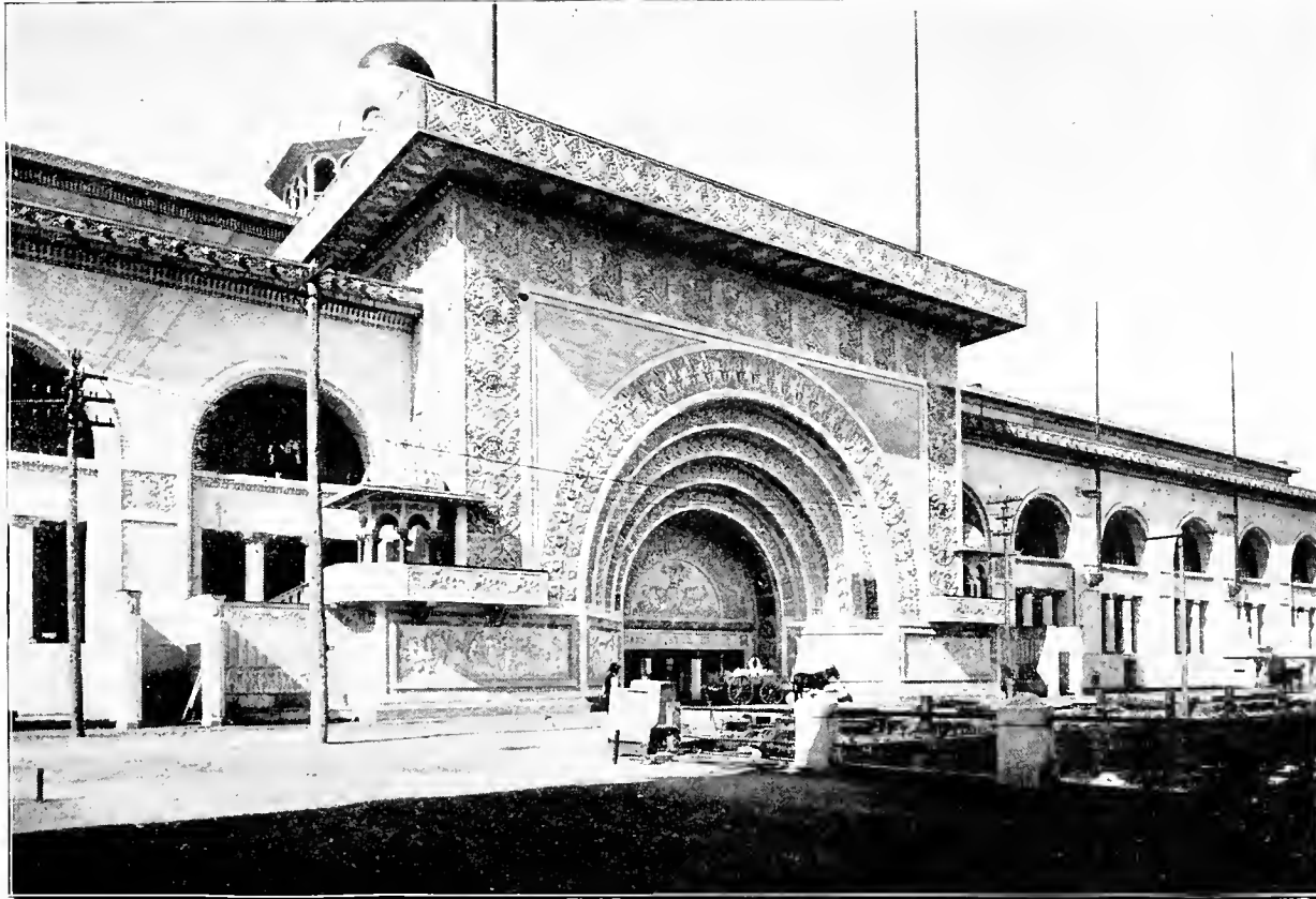
GOLDEN PORTALS. — The Main Entrance of "Transportation Building." This entrance is a series of receding arches, with bas-reliefs on either side and over the inner door. The entire surface is treated with gold leaf which gives a brilliant and imposing effect. The designs are emblematic of the various aspects of Transportation from earliest days to modern times. The elaborate carvings and mural paintings are a fascinating and instructive study in themselves.
