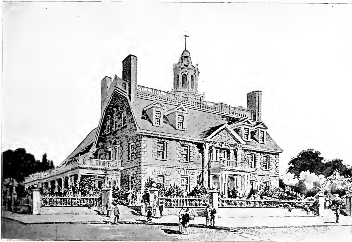
MASSACHUSETTS STATE BUILDING. -- Designed by Peabody & Stearns of Boston. It is 84x 91; cost $50,000. It is a reproduction of the old "Governor Hancock" house of colonial days, which stood on Beacon Hill in Boston, just West of the State House and facing the Common. The exterior is of "staff," marked and painted to represent granite. The main entrance is a huge mullioned door-way, in harmony with the whole effect. An interesting feature of the old "Bay State" headquarters is the old fashioned flower garden surrounding the building.
