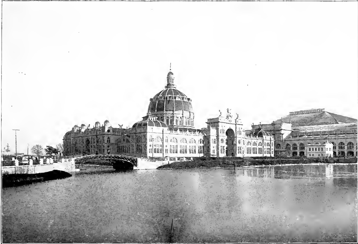
UNITED STATES GOVERNMENT BUILDING. — Designed by Mr. Windrin, succeeded by W. J. Edbrooke. It is 345x415; covers 3½ acres; cost $400,000. On the same island as the Building of Manufactures and Liberal Arts. Its dome, 120 feet in diameter, and 150 feet high, detracts from the general effect; but to the casual observer this may be lost sight of, for it contrasts well with the surroundings. Contains exhibits from Government Departments, — Post Office, Treasury, War, State, Interior, Fisheries, Smithsonian Institute, etc.
