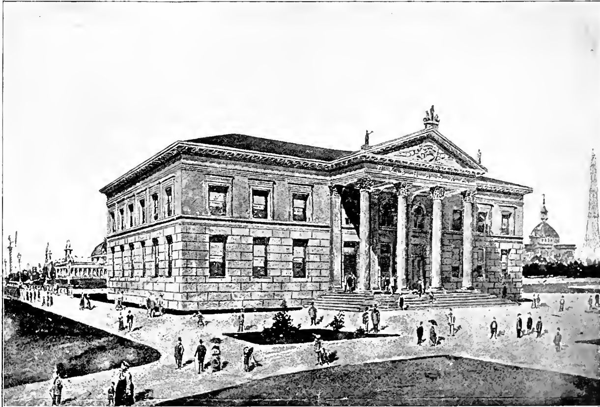
NEBRASKA STATE BUILDING. —Dimensions, 60x100: covers nearly 6,000 feet of ground: cost $15,000. Style of architecture, strictly classical, of the Corinthian order. Two stories high, with floor area of 12,000 square feet. East and West fronts have very wide porticoes supported by six massive columns 25 feet high. North of the magnificent "Art Palace."
