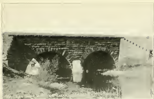
BRIDGE OVER DU PAGE RIVER, LOMBARD
