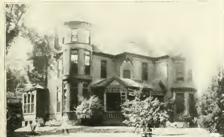
LIBRARY, HINSDALE— FORMERLY RESIDENCE OF D. K. PEARSONS
