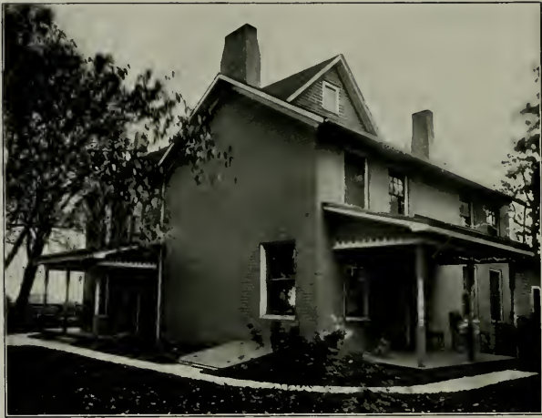
HOUSE BUILT BY FRANCIS WHITCOMB Still standing in Catlin
