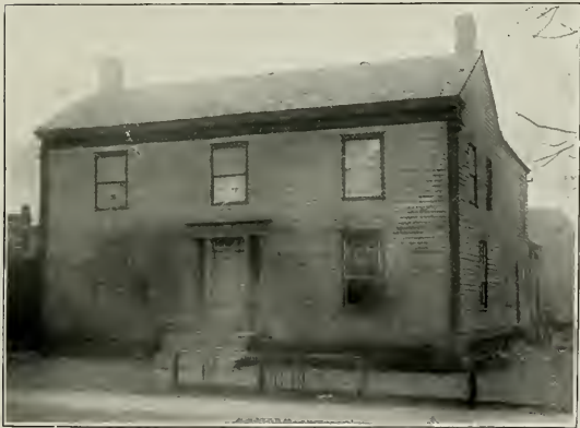
WILLIAM BANDY HOUSE ON EAST NORTH STREET
