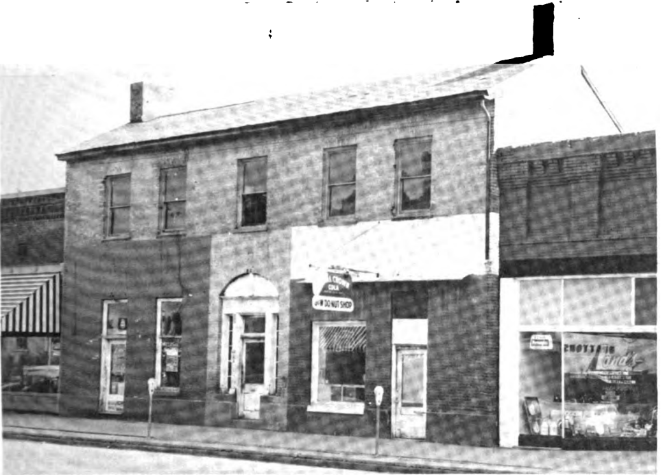
Neglected, abused, dilapidated, 132-year-old Ratcliff Inn looked like this in 1960 when the White County Historical Society saved it from destruction, purchased and restored it. The inn was built in 1828 by James Ratcliff.
