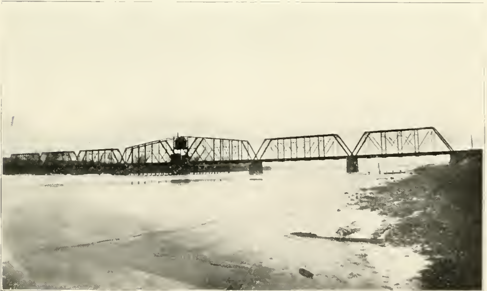
THE PEORIA & PEKIN UNION RAILROAD BRIDGE, RECENTLY SUPPLANTED BY A FIVE HUNDRED THOUSAND DOLLAR STRUCTURE
