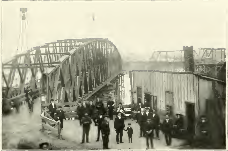
SCENE AT COLE BRIDGE, FOOT OF BRIDGE STREET, JUST BEFORE BRIDGE WAS TORN DOWN IN 1908 FOR NEW STRUCTURE The bridge "crowd" say "good-bye"
