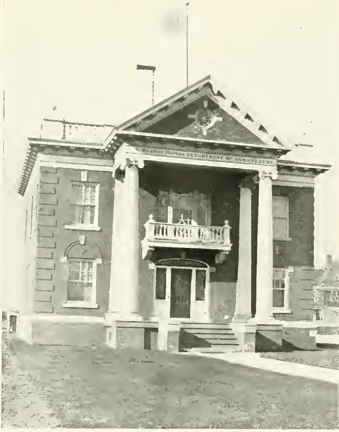
U. S. WEATHER BUREAU STATION
