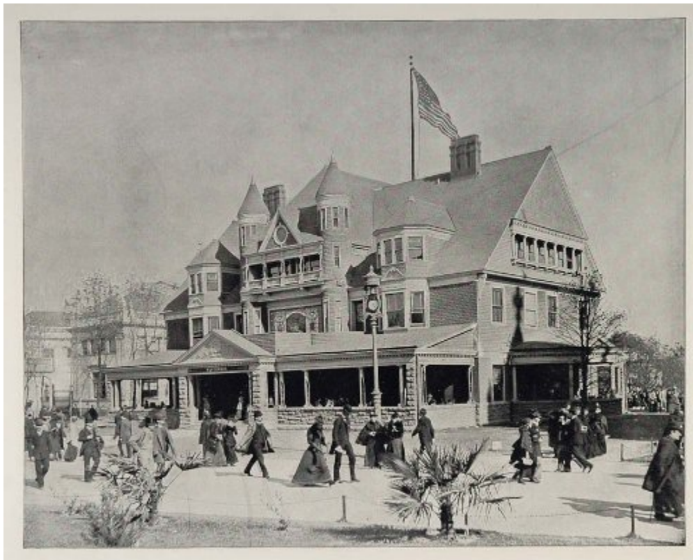
Wisconsin State Building
