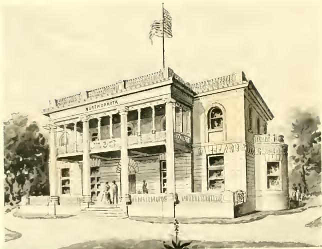
NORTH DAKOTA STATE BUILDING 70 x 40 feet. Cost, $11,000.
