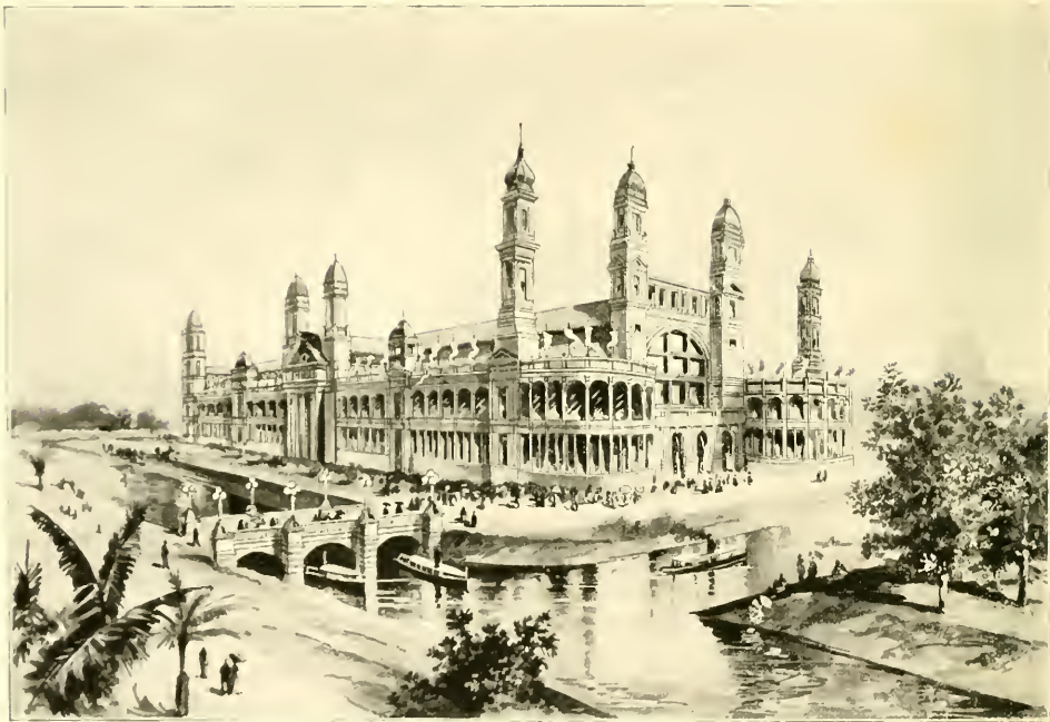
THE ELECTRICAL BUILDING.
