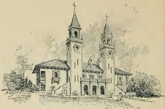
THE COLORADO STATE BUILDING.
