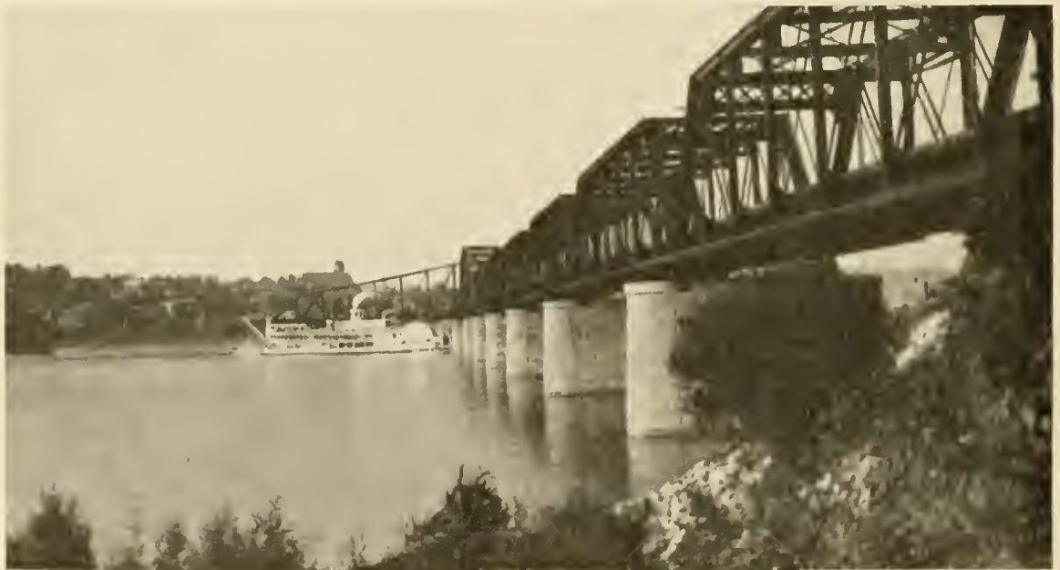
THE "BURLINGTON" BRIDGE AT ALTON.
