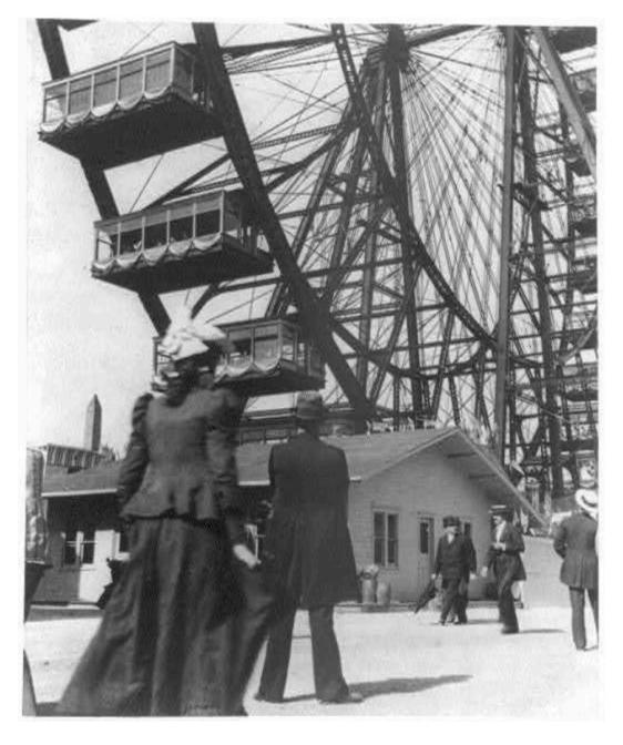
Each car weighed 13 tons. Stepped platforms at the base of the Wheel enabled six cars to be loaded and unloaded at a time. Fully loaded, the Wheel's maximum capacity was an astounding 2160 passengers. Each car carried an employee to keep an eye on the passengers' health and wellbeing. Fainting was a problem considering the thin-waist fashion for women at that time.
