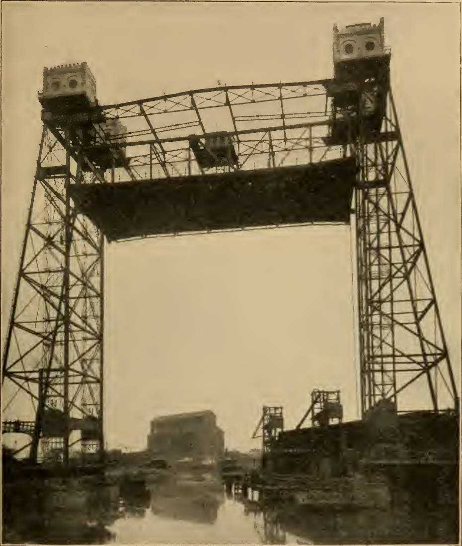
VERTICAL LIFT BRIDGE, HALSTED STREET
