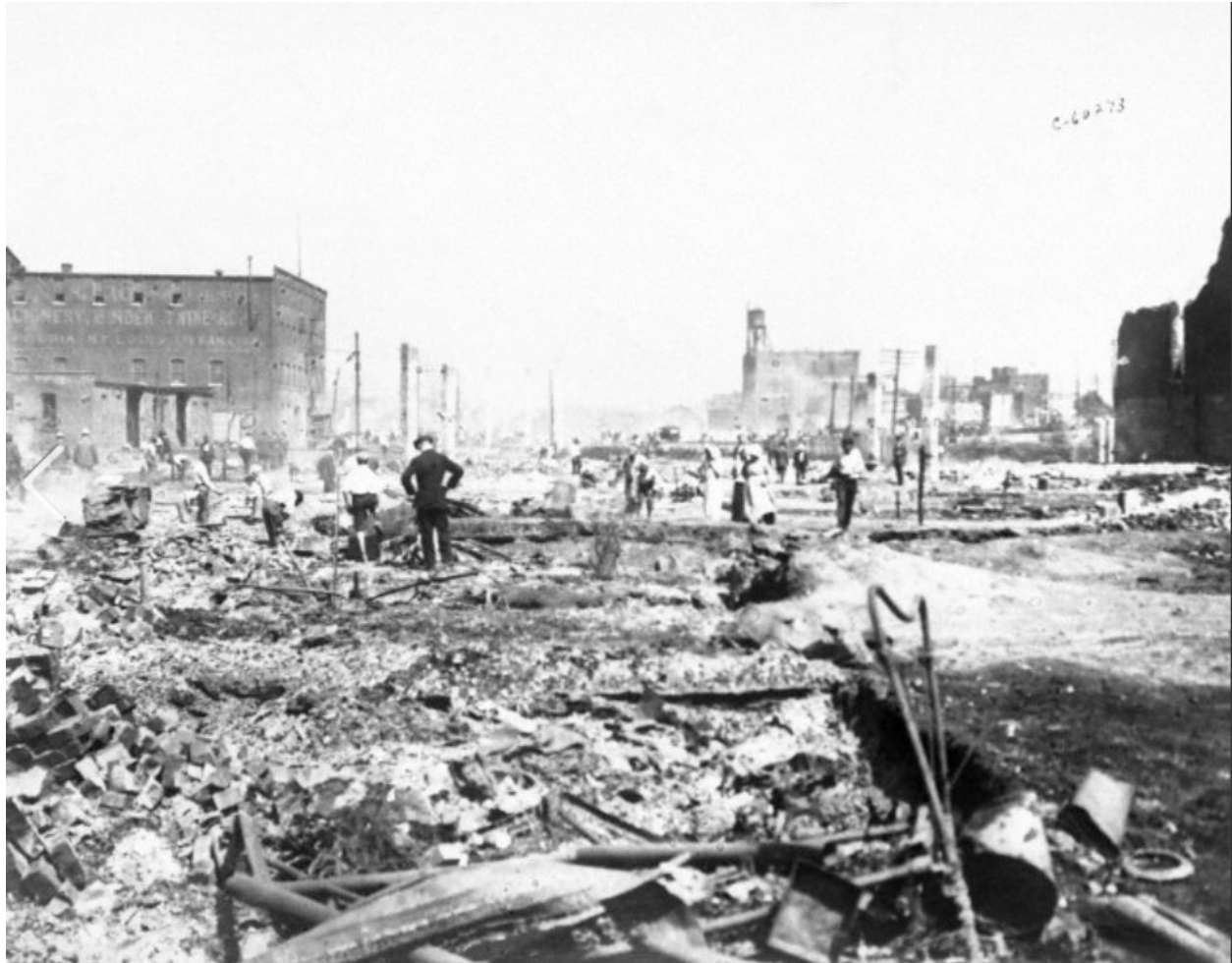
Six blocks of Walnut Street reduced to rubble from fires started during racially motivated riots in East St. Louis, IL.
