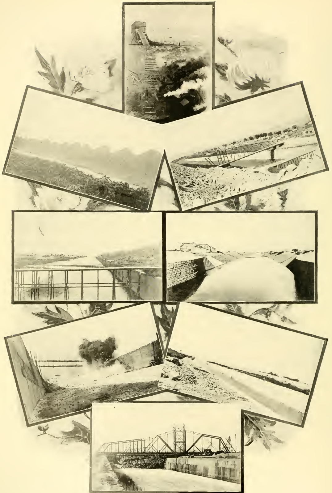
VIEWS OF DRAINAGE CANAL.
