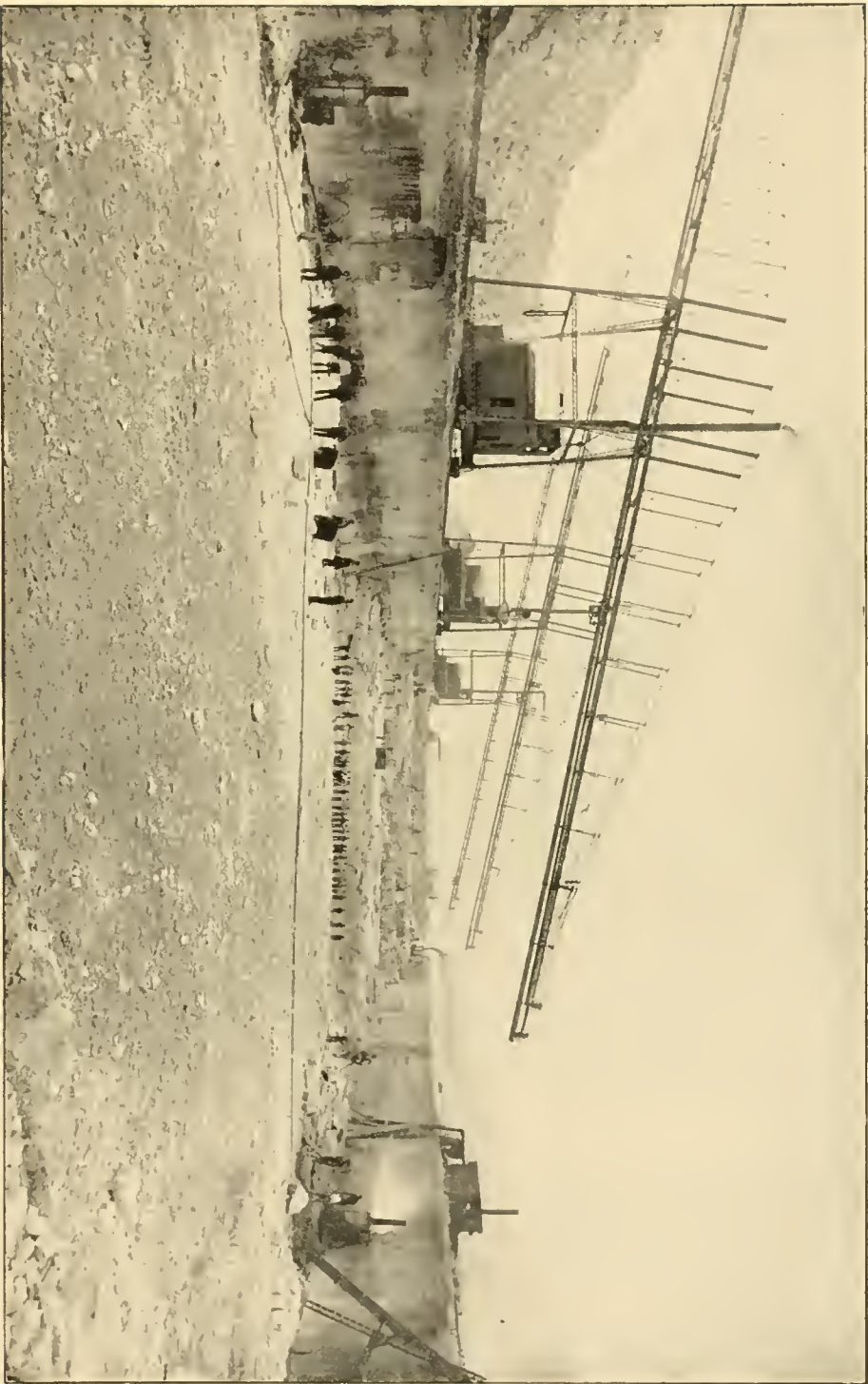
EXCAVATION IN ROCK FOR DRAINAGE CHANNEL AND WATERWAY. (FILL DEPTH IN CENTER.)
