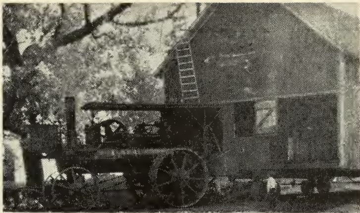
Gaare barn moved in approximately 1916. Building pulled by steam engine and loaded on 8 wood wheels.
