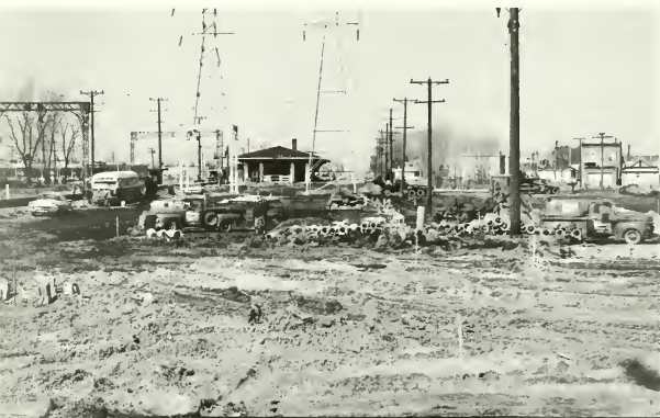
By March 1964, the Park'n'Ride lot contractor had completed rough grading and was installing the drainage system. Early spring snow then made paving work impossible for several weeks.
