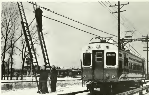
Signal, communication and station lighting cables were being installed while the first test run of car #1 through to Dempster was being made on March 30, 1964.
