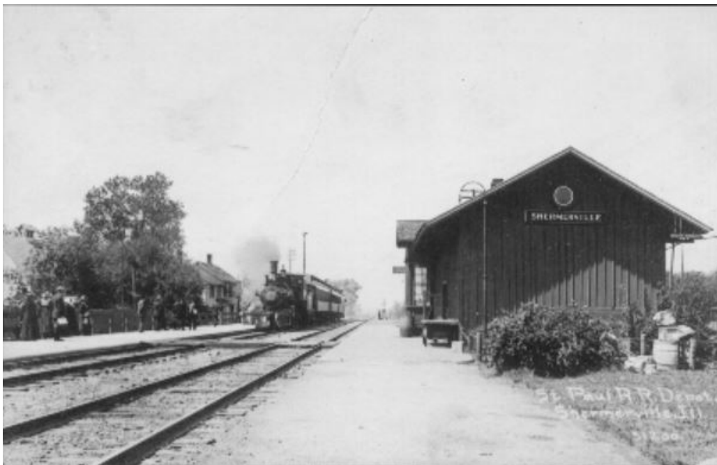
The train depot was located across the tracks from the present station. The one on the left was replaced by the Landwehr Building. (1914)
