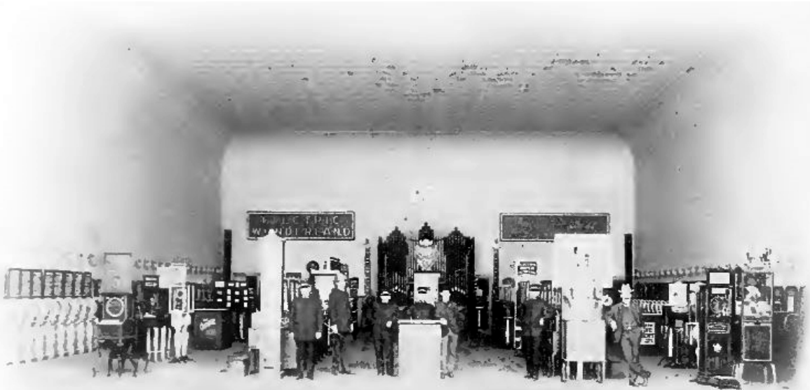
Interior View of the Automatic Vaudeville
