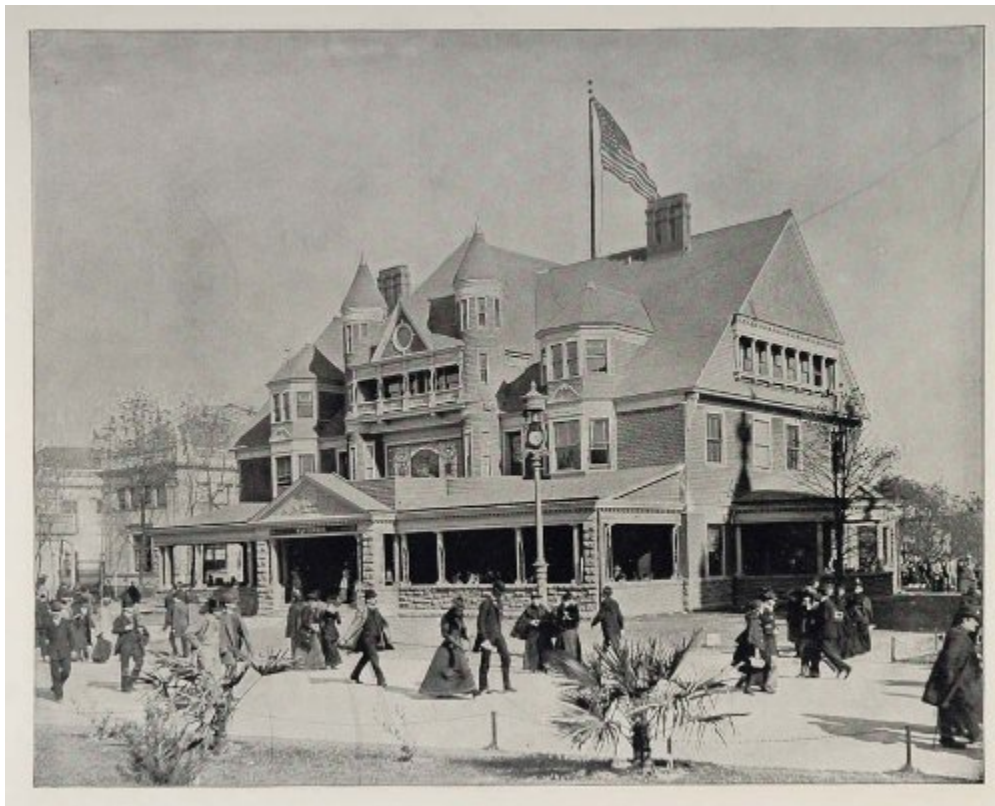
Wisconsin State Building
