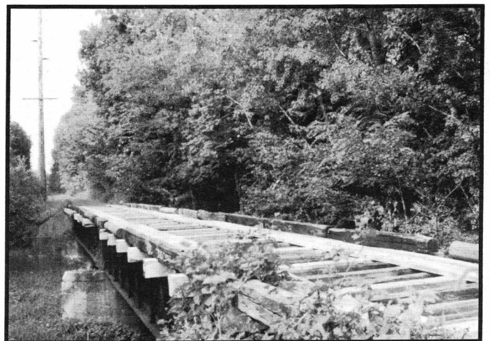
#7 Looking at it to the North.
