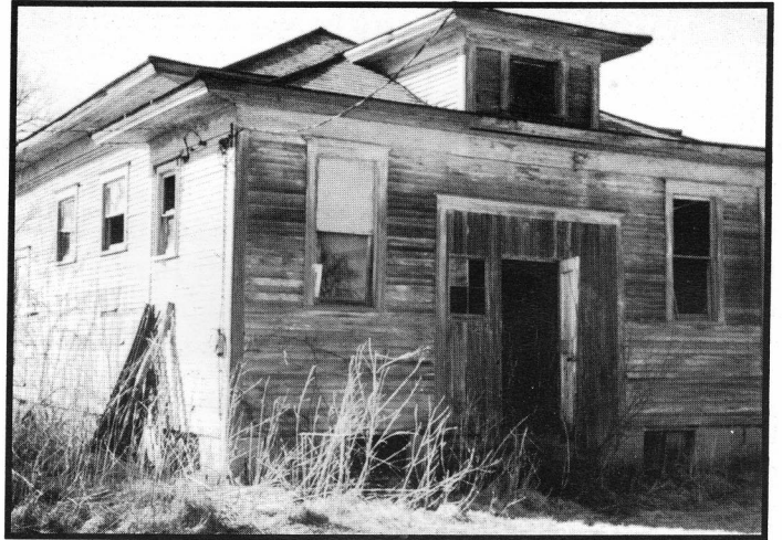
An original schoolhouse in Cayuga burned down about a year ago.
