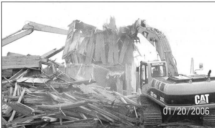
Here you can see the high hoes crushing one of the bins after it is on its side.
