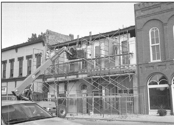
The bricks in the Downey Building were removed one by one by the workmen of Parks Construction, the Atlanta-based contractor doing Phase I work on the Palms Grill Cafe Project.
