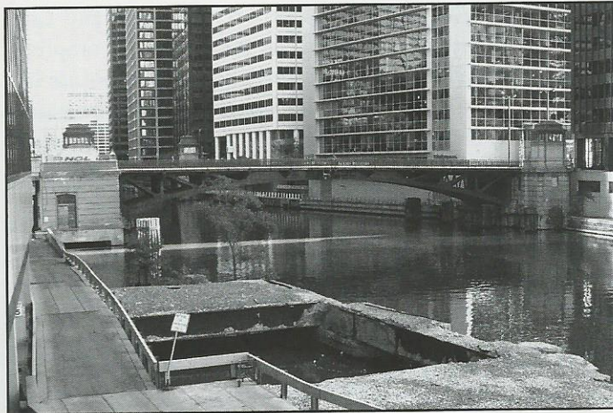
Looking north at the Jackson Boulevard Bridge, currently closed to traffic due to construction on the approach viaduct to the west. In the left foreground is the remnant of the Jack Knife Bridge pier.
