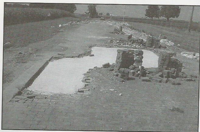
You can see the depth of the repair of the brick road
